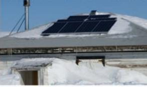
This ranger's cabin on Herschel Island, Yukon, has solar panels on its roof.
